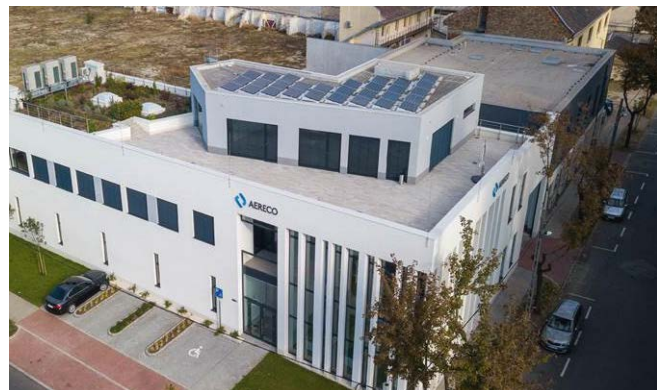
Solar panels installed on site in Hungary
